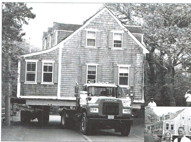
The historic home, previously one of the Three Sisters overlooking Stage Harbor, crept along Champlain Road to its new home on Sears Road.
