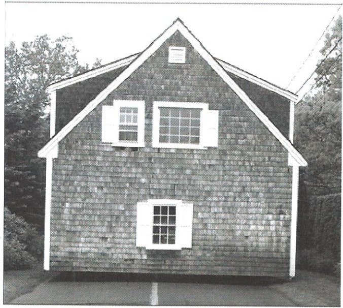
A garage salvaged from one of the other Three Sisters homes, a 1940 Cape, was also moved and will be attached to the 1762 house at its new site.
